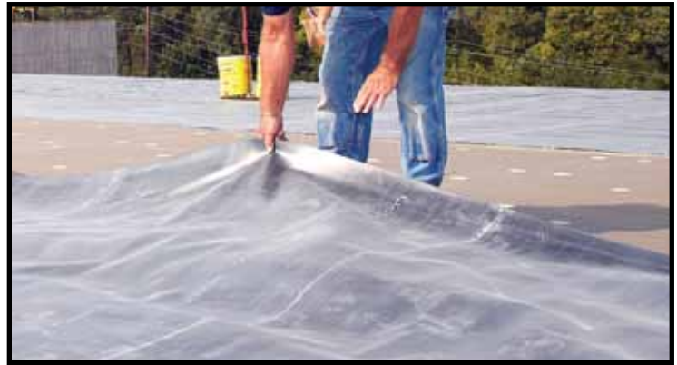
Mule-Hide Pre-Taped EPDM wide-width sheeting features a single-fold sheet.
