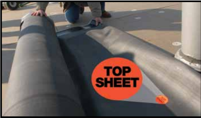
To ensure correct roll-out, locate the orange "TOP SHEET" sticker on 2-Packs.
