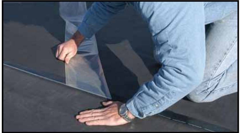
Mule-Hide Pre-Taped EPDM makes wrinkle-free seaming easier.
